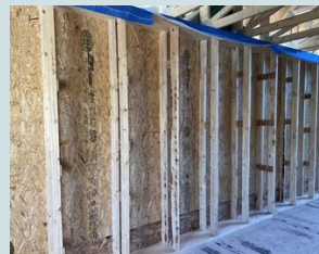
CELLULOSE IN TIMBER FRAME
