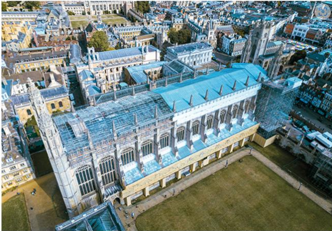
Figure 6. The shallow 25° roof pitch meant that the north and south slopes were suitable for PVs. Source: Cibsejournal.com
