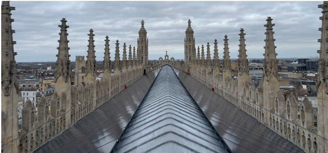
Figure 5. The panels are part of the renovation of the 1950s lead roof of the Chapel, which was no longer watertight. Source: Maxfordham.com,
