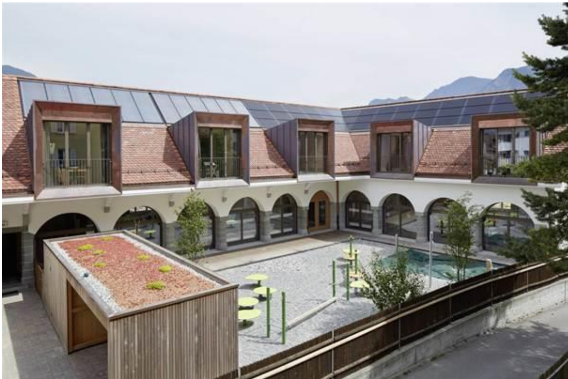
Figure 15. The roofs of the annex buildings have been remodelled incorporating solar thermal and PV panels and the volume extended with 5 large dormer windows. Source: hiberatlas.eurac.edu
