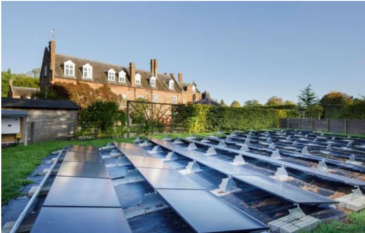
Figure 13. Alternative view showing the screening, PV panels and supporting framework. Source: Historic England
