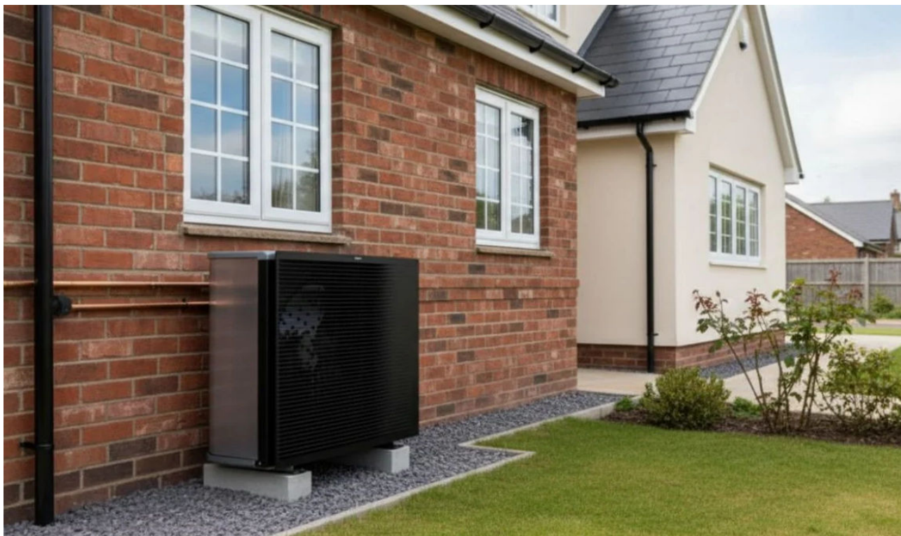
Heat pump installations can impact the character of a building, but there are strategies to minimise the impact.
